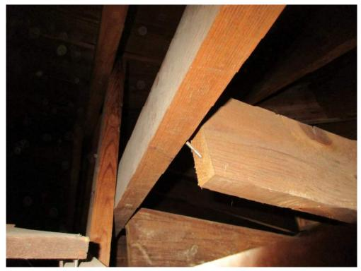
Photo 15: Typical Nail Pullout at Inadequate Roof Framing Connection
