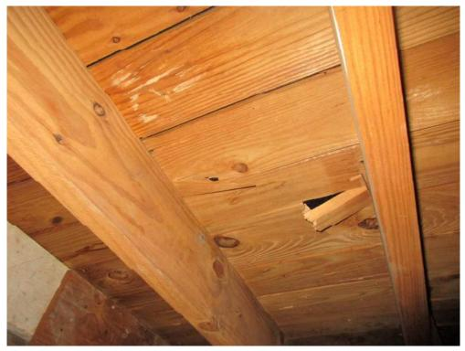
Photo 27: Typical Cracked and Damaged Roof Decking
