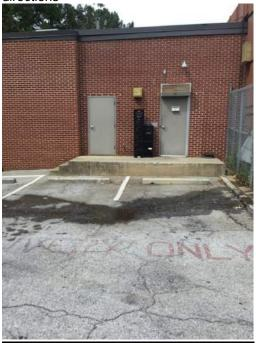
**Description:** Existing loading dock doesn't have handrails along stairs
