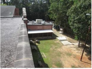
**Description:** Existing wood framed canopy was originally installed for temporary portables during previous construction and is no longer needed. The frame is also no longer structurally sound.
