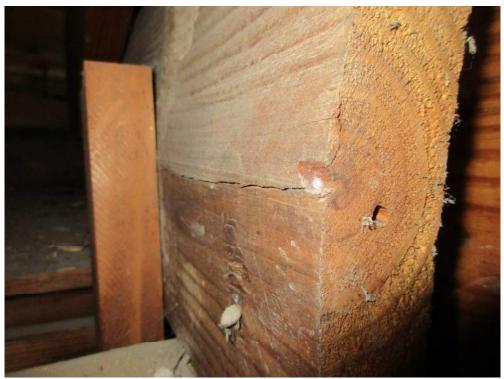
Photo 20: Cracked Pre-1949 Roof Rafter-to-Exterior Wall Connection
