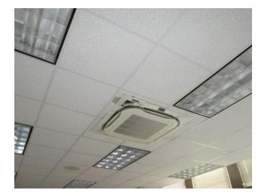
**Description:** Several fan coil units have been damaged. Covers and filters are missing
