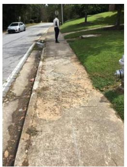
**Description:** Section of concrete walk needs to be repaired along roadway
