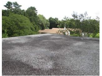
**Description:** Built-up & ballasted roof areas that are retaining moisture.
