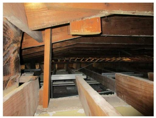
Photo 17: Removed Bearing Member at Pre-1949 Roof Structure
