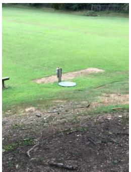
**Description:** According to Assessment report existing sewer system was installed in 1940 with 50 year service life. According to the achieved survey from 1991 the existing sewer line is 8" clay pipe. At time of visit we observed what appears to be a lift station down in field. This life station most likely pumps the building sewer flows around the existing building to the existing sewer system in the r/w
