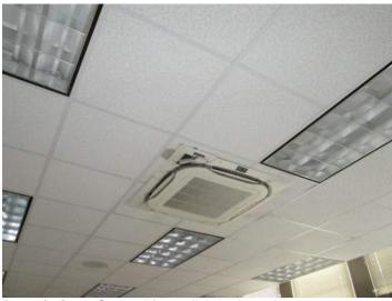
**Description:** Several fan coil units have been damaged. Covers and filters are missing
