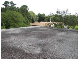
**Description:** Built-up & ballasted roof areas that are retaining moisture.
