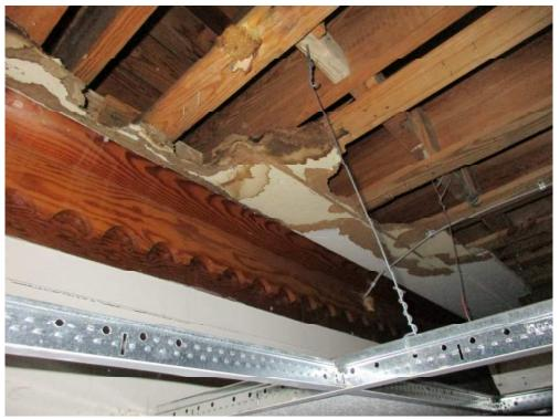
Photo 24: Water Damage at 1949 Roof Structure and Ceiling at the Northeast Classroom North Wall
