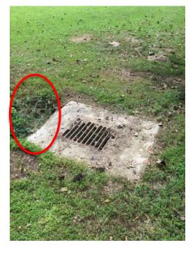
$\underline{\textbf{Description:}}$  Erosion in courtyard and damaged yard drain
