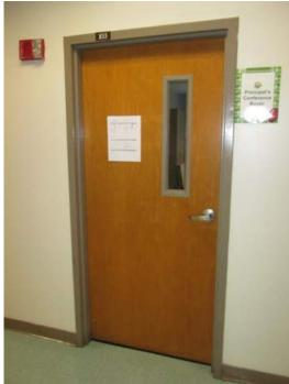
**Description:** Existing solid wood doors and door hardware throughout the facility appears to be functioning properly. The existing classroom locks are not up to date with the latest lockdown procedures.
