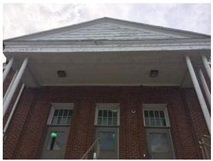
**Description:** The majority of the wood trim and soffits of Buildings #2031 and #2030 is deteriorating and in need of repair.
