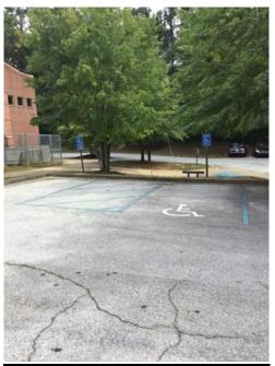
**Description:** ADA striping not compliant with code. The 3<sup>rd</sup> ADA space needs to have a striped landing and doesn't appear to be less than 2% slope in all directions
