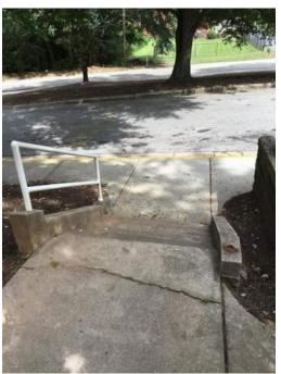
**Description:** Concrete steps missing handrail and side walk is cracked
