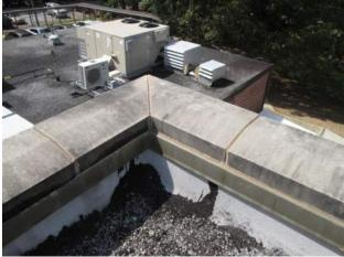
**Description:** Existing stone parapet cap appears to be needing cleaning.
