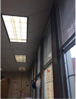
**Description:** Windows at second floor of Building #2030 are splaying outward and do not have adequate support between windows.
