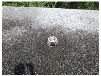
**Description:** Existing roof drains appear in fair condition and no clogging was observed.
