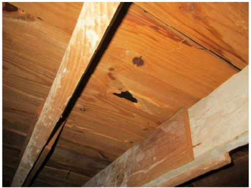
Photo 28: Typical Cracked and Damaged Roof Decking
