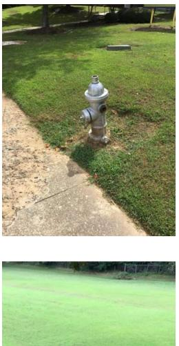
**Description:** According to Assessment report existing water line was installed in 1940 with 50 year service life. Was only able to locate one (1) hydrant on site which is in the front of school in r/w
