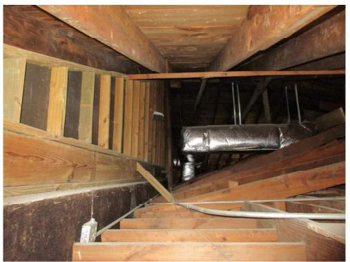
Photo 4: End Wall 2x Truss Structure at Southern Expansion Joint (North Edge of 1999 Addition)
