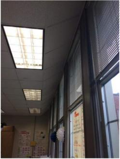
**Description:** Windows at second floor of Building #2030 are splaying outward and do not have adequate support between windows.
