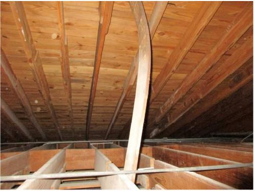
Photo 18: Water Damage and Roof "Sagging" Causing Excessive Bending of 1949 Roof Structure Bracing
