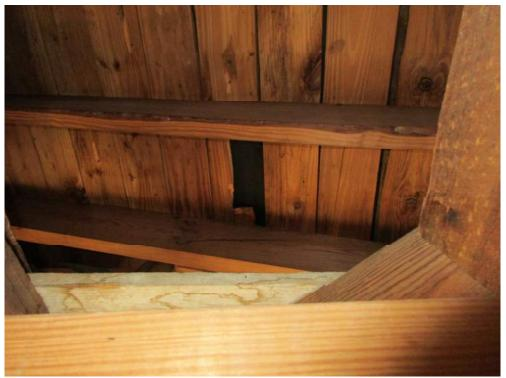
Photo 26: Typical Cracked and Damaged Roof Decking
