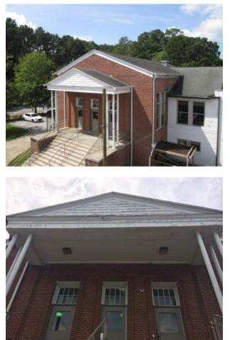
**Description:** The majority of the wood trim and soffits of Buildings #2031 and #2030 is deteriorating and in need of repair.
