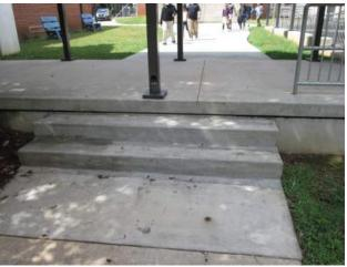
**Description:** Exterior stairs missing railings. **Recommendation:** Install handrails.
