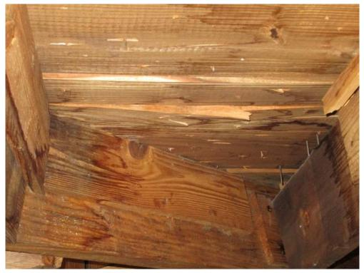
Photo 25: Typical Cracked and Damaged Roof Decking
