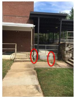
**Description:** Erosion in courtyard and damaged yard drain
