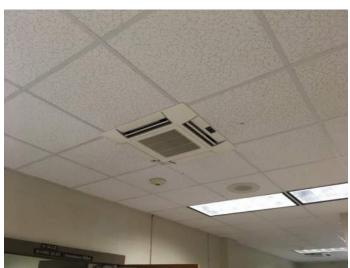
**Description:** Existing HVAC system is VRF with dedicated outdoor air units. Dedicated split system fan coil units are provided for IT/Data rooms. A new building automation system was also provided.
