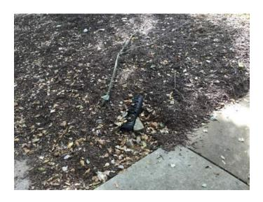
**Description:** HDPE drainage pipe daylighting out of grade destroyed
