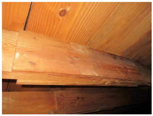
Photo 13: Typical Pre-1949 Roof Structure Damaged Rafter Splice
