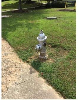
**Description:** According to Assessment report existing water line was installed in 1940 with 50 year service life. Was only able to locate one (1) hydrant on site which is in the front of school in r/w
