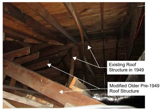
Photo 1: Existing Pre-1949 Roof Structure Additions
