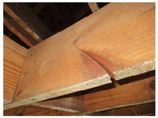
Photo 29: Typical Cracked Ceiling Joist
