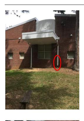
Description: Downspout damaged
