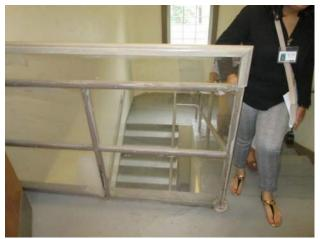
**Description:** Railings in existing typical exit stair do not meet current Life Safety codes.
