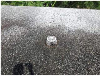
**Description:** Existing roof drains appear in fair condition and no clogging was observed.
