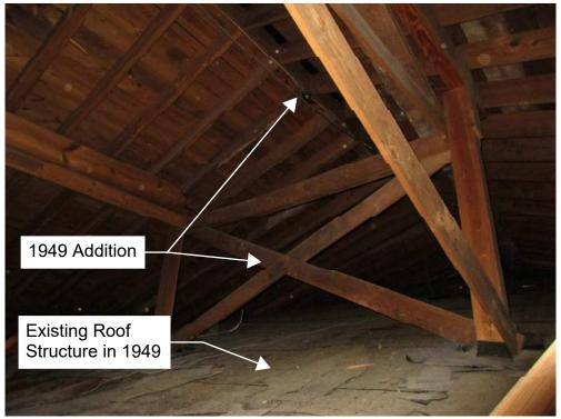
Photo 2: Existing 1949 Roof Structure Addition Built Atop Pre-1949 Structure (Looking South From Northwest Classroom)
