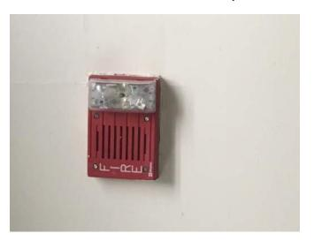
The existing fire alarm system does not meet current code. In some areas it appears fire alarm devices have been removed. A new fire alarm system should be provided to meet code.
