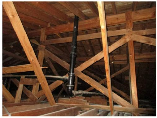
Photo 11: Typical 1949 Roof Structure Lateral Bracing, Diagonal, and Kicker System
