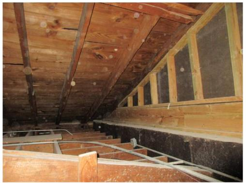
Photo 10: End Wall 2x Truss Structure at Southern Expansion Joint (North Edge of 1999 Addition)
